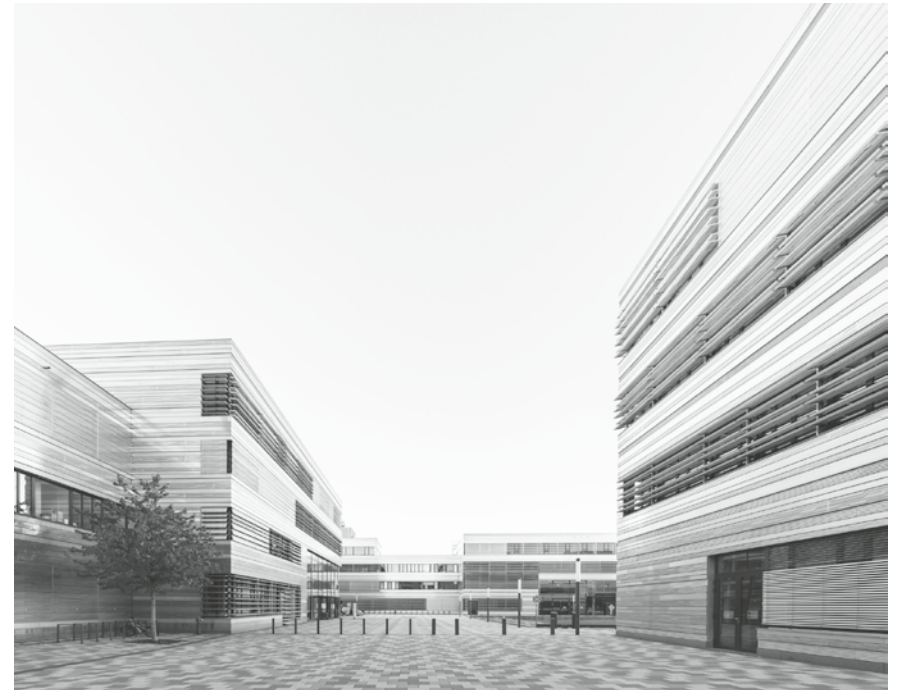
HSD Campus Derendorf, exterior view
